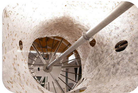
Figure3: The pavilion in the process of weaving by a living organism digitally controlled by humans
